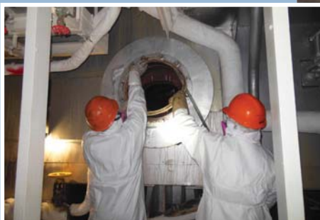
Removal of asbestos flanges
